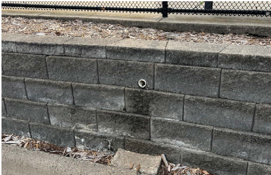
Deck Drain Outfall
