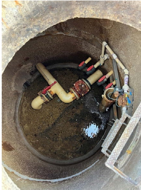
Interior of Pool Surge Tank
