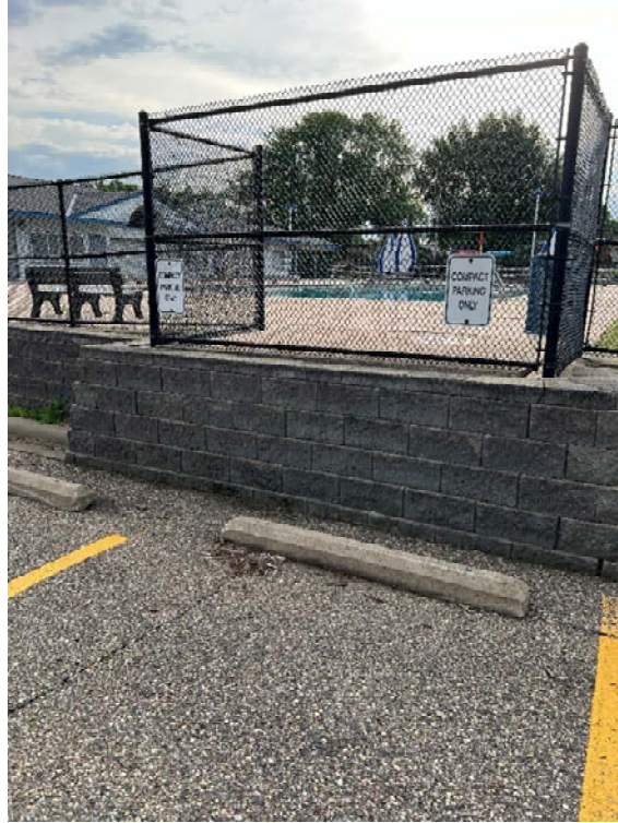
Facility Site Enclosure and Foundation Wall
